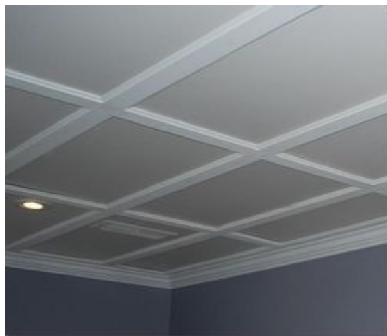
Figure 2. Fall ceiling made of Plaster of Paris
